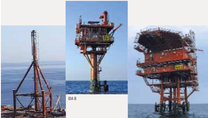
JACKET UNDER CONSTRUCTION
